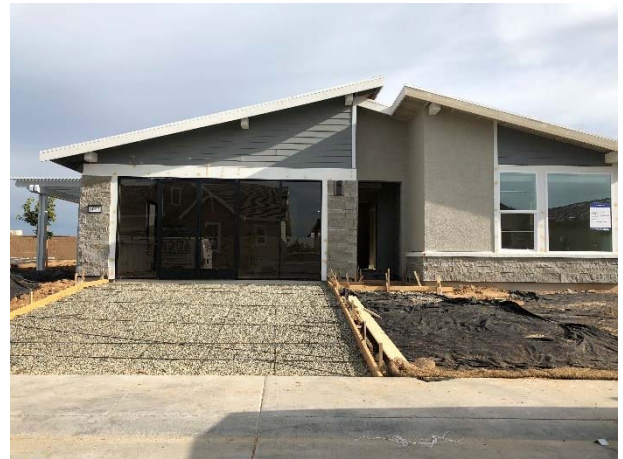
Lennar model homes under construction
