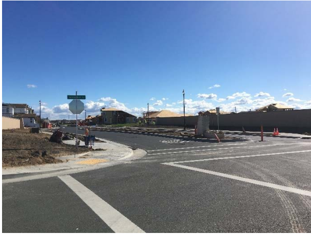
Taylor Morrison homes under construction
