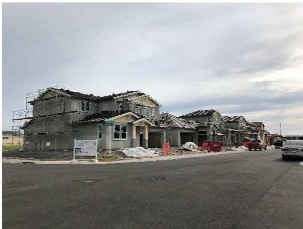
Lennar model homes under construction
