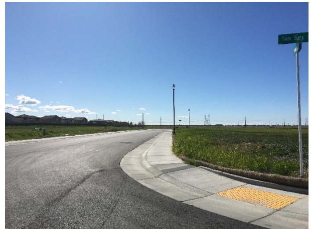
Finished lots/homes under construction
