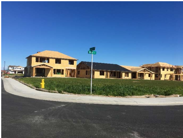
Finished lots/homes under construction
