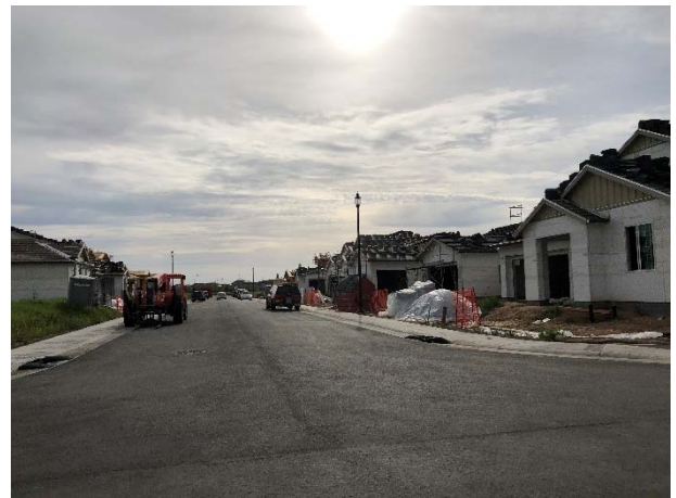
Lennar model homes under construction
