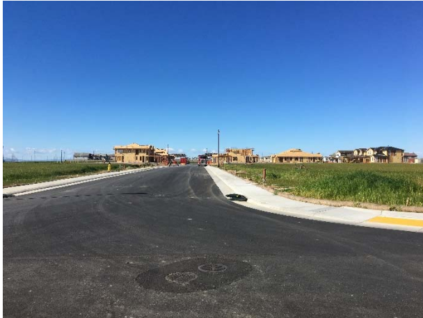
Finished lots/homes under construction
