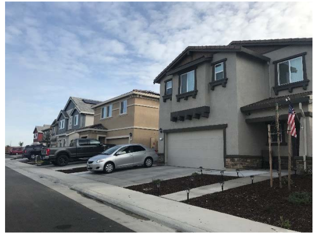
Completed Homes in Manchester Development
