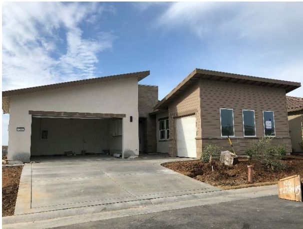
Lennar model homes under construction
