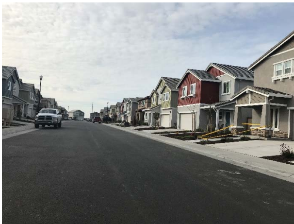
Completed Homes in Manchester Development
