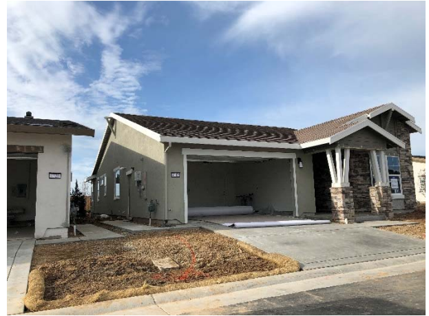
Lennar model homes under construction
