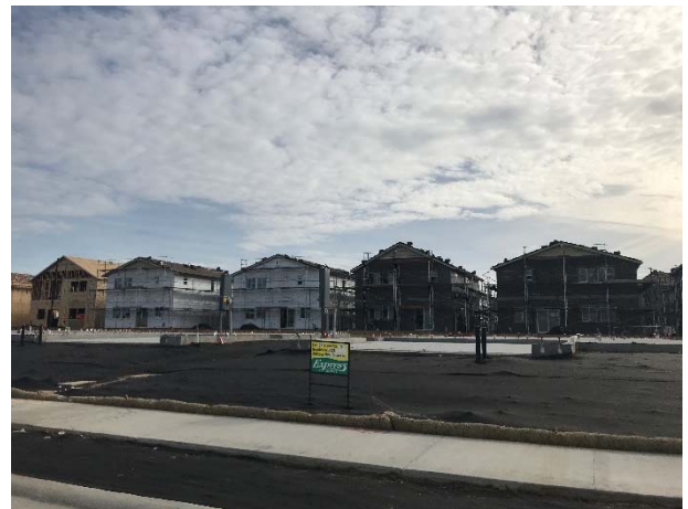
Completed Homes in Manchester Development
