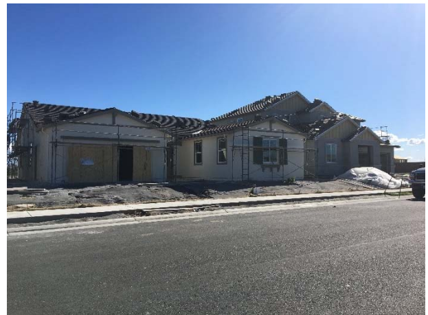
Taylor Morrison models under construction
