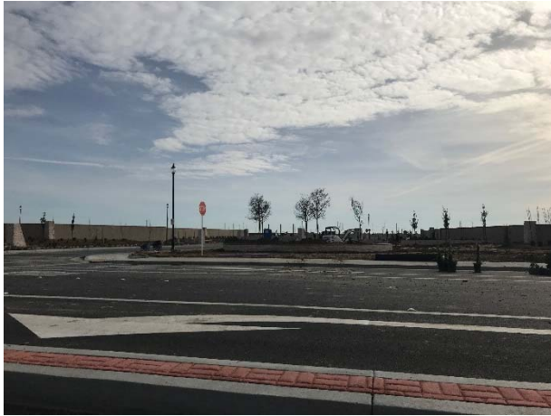
View of Lennar project from Pleasant Grove Boulevard
