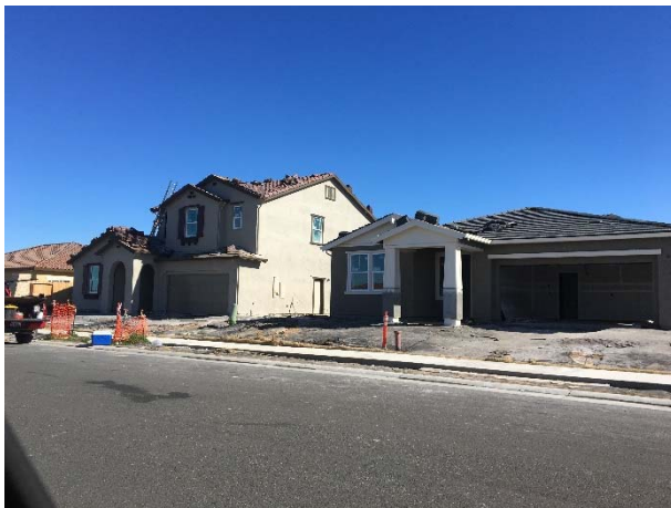
Taylor Morrison models under construction
