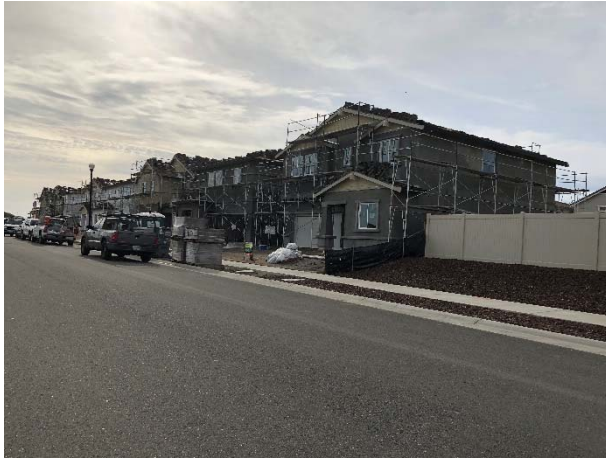
Lennar model homes under construction
