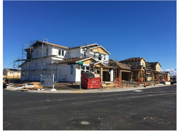
Taylor Morrison homes under construction
