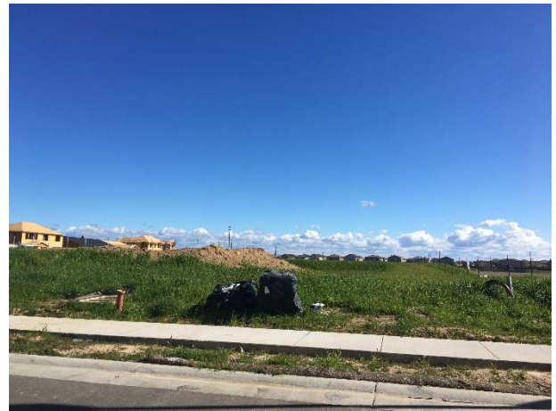
Finished lots/homes under construction
