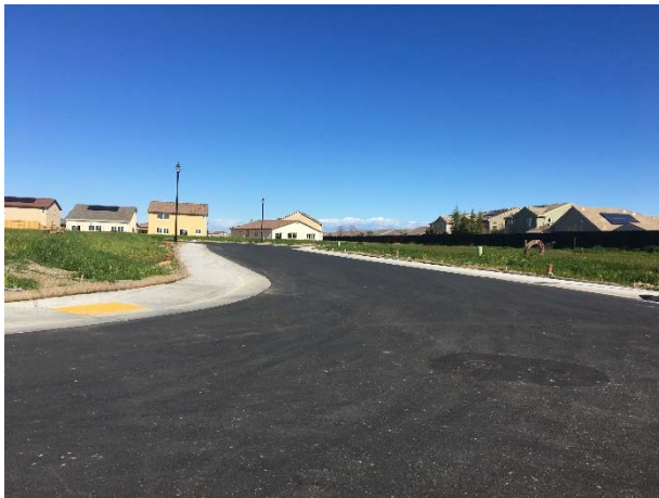
Finished lots/homes under construction
