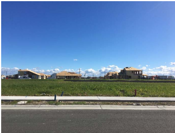
Finished lots/homes under construction
