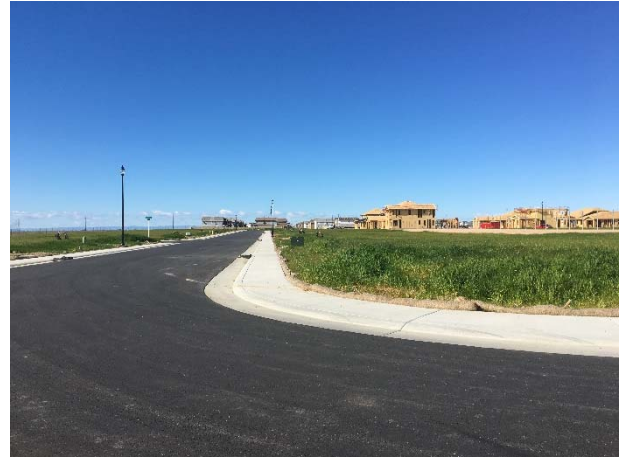
Finished lots/homes under construction
